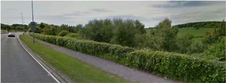
FIG 3 Existing woodland and hedging along A92 Road.
